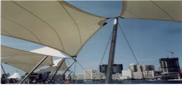
1. Shade canopies, Dubai, UAE
