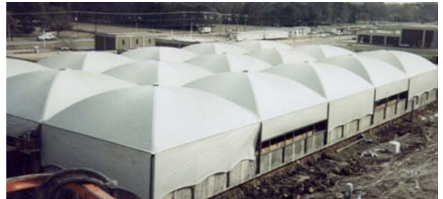
10. Water treatment plant, Chesapeake, VA
